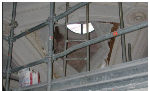
Figure 7 - Opening of the six pentagons located in the dome above the altar after the untap the paint surface
